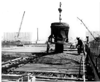
Pouring the concrete floor for the VAB.
